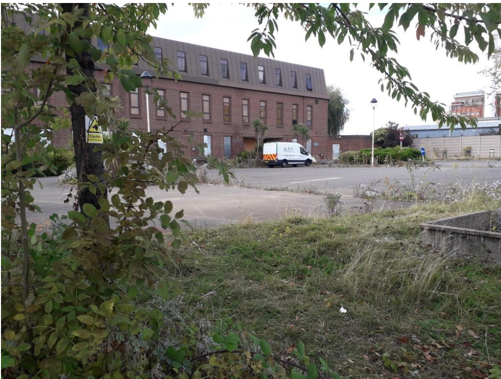
Elevation from the existing access Road
